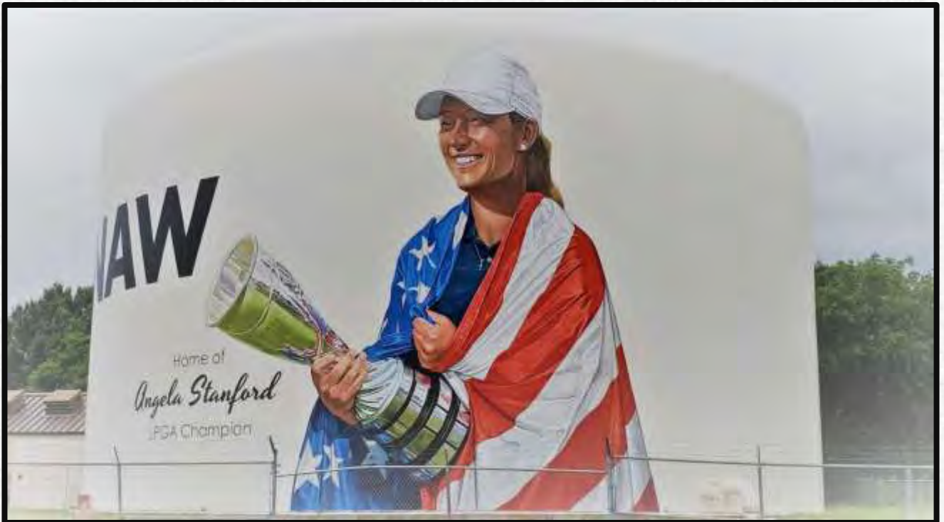
Above ground fresh-water tank in Willow Creek Park
